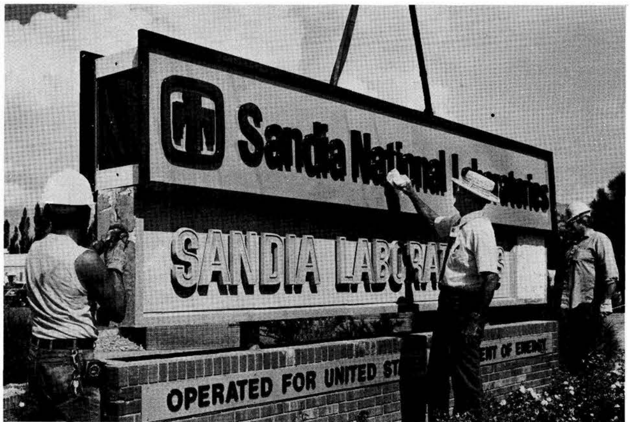
NEXT TIME you're driving on Wyoming west of Bldg. 800, check out the new sign (here getting a dusting by Ward Hunnicutt, Director of Plant Engineering 7800). The new sign, slipped into place over the old one, is a scaled-up replication of Sandia's official logo.
